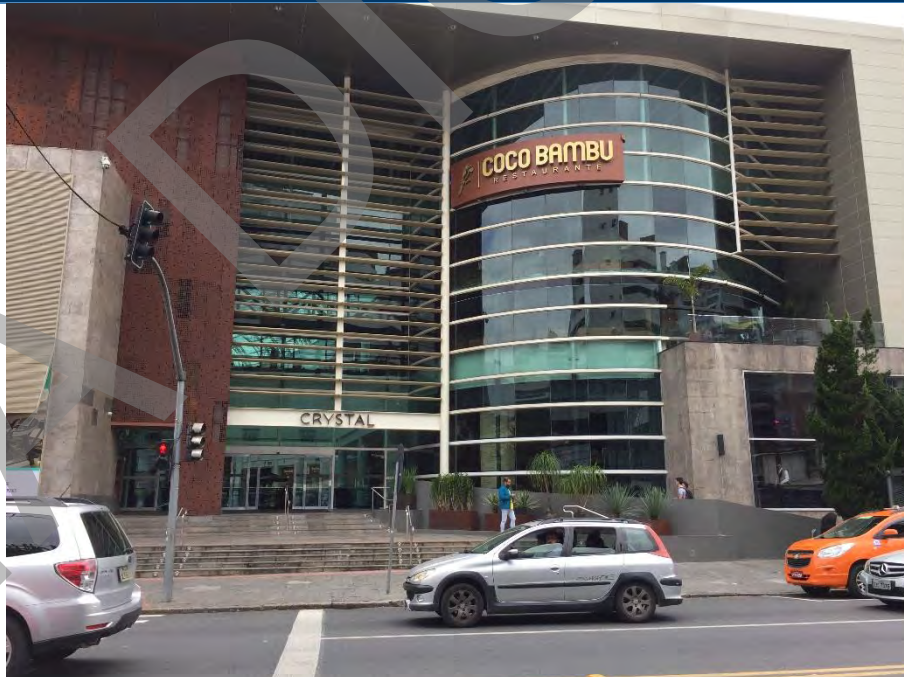
VIEW OF THE SHOPPING CENTER FAÇADE
