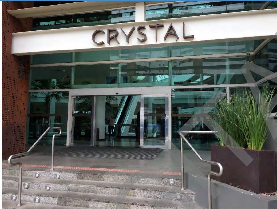
VIEW OF THE SHOPPING CENTER FAÇADE
